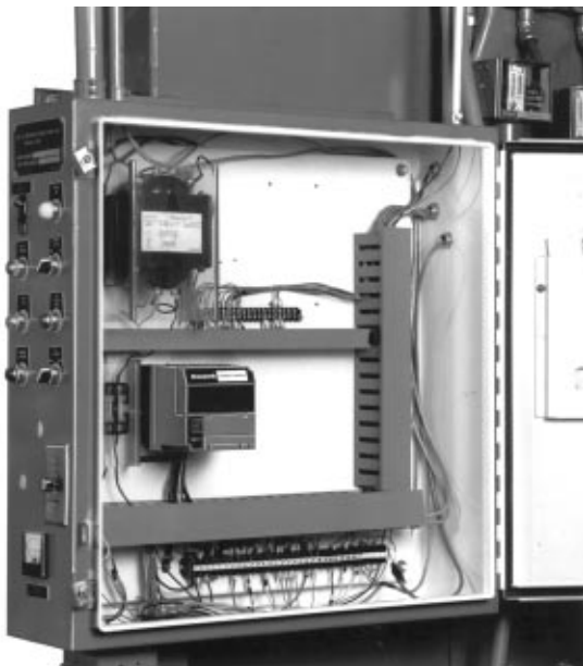
Fig. 7. Electrical panel installation.
